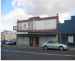
763-765 High Street, Reservoir
