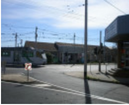
East Preston Tram Depot, 211-243 Plenty Road
