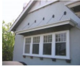
16 Spencer Street: Window and Hood Detail
