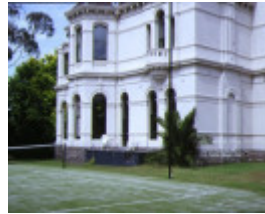
myoora alma road caulfield rear view
