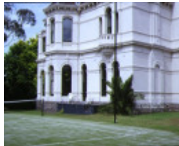
myoora alma road caulfield rear view
