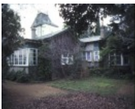
halstead caufield view of house jul1978
