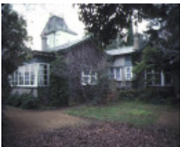
halstead caufield view of house jul1978
