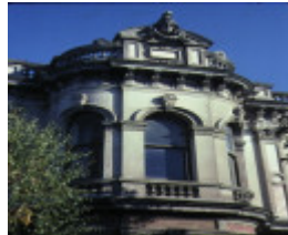
labassa caulfield external windows
