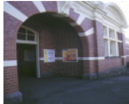
caulfield railway station normanby road caufield side detail jan1998
