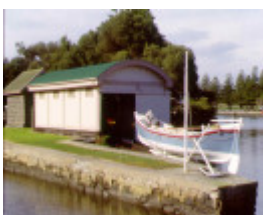
1 lifeboat station port fairy sw aug1999
