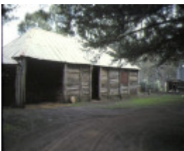
glenisl homestead glenisl via cavendish outbuilding jul1978
