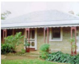
neuchatel merrawarp road ceres verandah view publication
