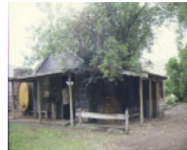
neuchatel merrawarp road ceres outbuilding winery
