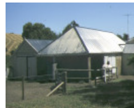
neuchatel merrawarp road ceres stables
