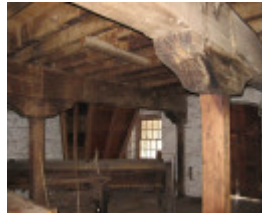
Mill interior Aug 2009
