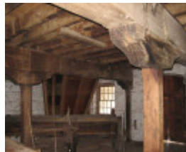
Mill interior Aug 2009
