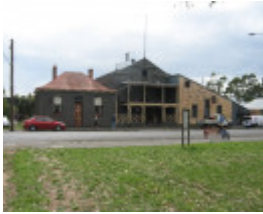
Piper Street view of the complex March 2010
