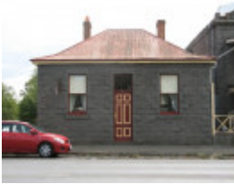
Street facade of residence March 2010
