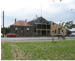
Piper Street view of the complex March 2010
