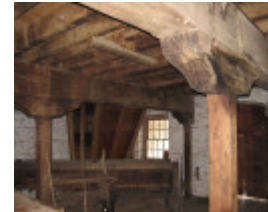
Mill interior Aug 2009
