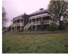
1 montpellier flour mill house calder hwy carlsruhe side view
