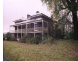
Montpellier Flour Mill House Calder Hwy Carlsruhe Front View
