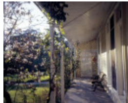
h01179 pastoria homestead baynton rd kyneton verandah she project 2003
