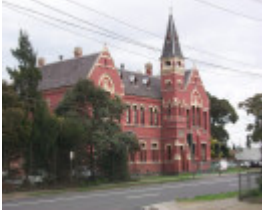
28247 Francis St Former Yarraville Primary School
