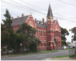
28247 Francis St Former Yarraville Primary School
