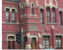
28247 Francis St Former Yarraville Primary School
