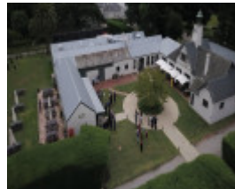
2015 stable yard with stables at centre with slate roof motor house with bell tower and 2015 additions
