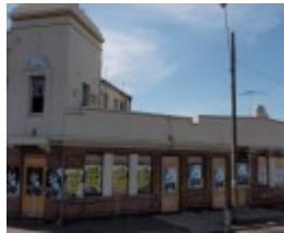
HO40 (2) - Rising Sun Hotel, 193 Geelong Road, Footscray.JPG
