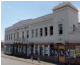
HO40 (1) - Rising Sun Hotel, 193 Geelong Road, Footscray.JPG
