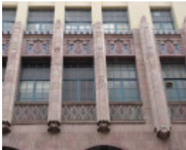
DJs former Coles_rear facade detail_16 Jan 08
