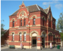
PARKVILLE POST OFFICE AND QUARTERS SOHE 2008
