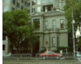
1 former residence 61 spring street july01
