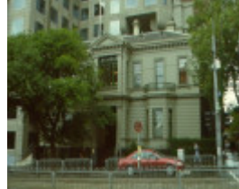
1 former residence 61 spring street july01
