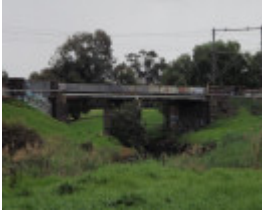
HO126 - Stony Creek Rail Bridge, Francis Street, Yarraville.JPG
