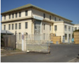
HO130 - Yarraville SEC Terminal Station, 308 Hyde Street, Yarraville.JPG
