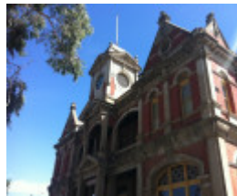
Before Photograph - Reference F3844 2014
