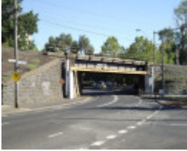
HO147 - Railway Bridge, Nicholson Street Rail overpass, Nicholson Street, Footscray.JPG
