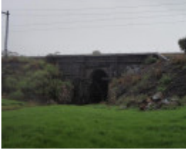
HO164(1) - Black Arch Bridge, Sunshine Rd, Sunshine.JPG
