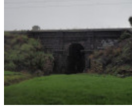
HO164(2) - Black Arch Bridge, Sunshine Rd, Sunshine.JPG
