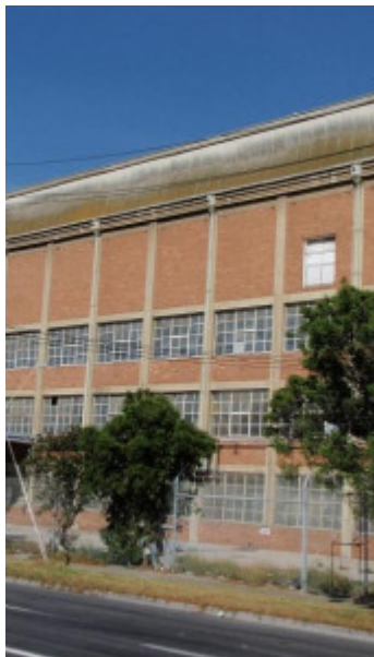
HO 160 (1) - Australian Estate Wool Store, 27-61 Sunshine Road, West Footscray.JPG
