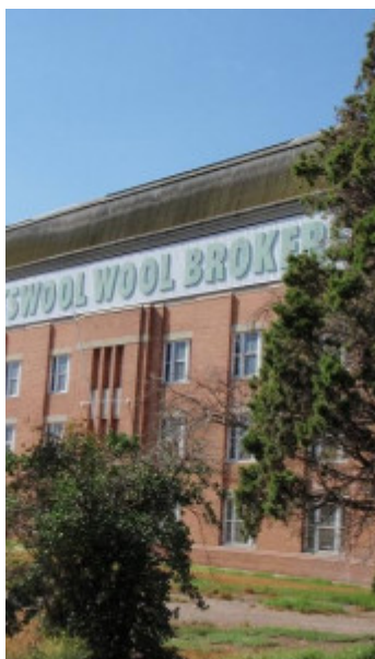
HO160 (2) - Australian Estate Wool Store, 47-61 Sunsiene Road, West Footscray.JPG
