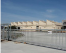
HO162 (1) - Olex Cables, 207 Sunshine Road, Tottenham.JPG
