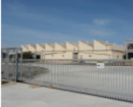
HO162 (1) - Olex Cables, 207 Sunshine Road, Tottenham.JPG
