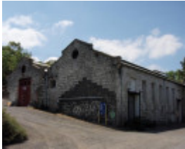
HO64(5) - Former Melbourne Meat Preserving Co. Pipemakers Park, Maribyrnong.JPG
