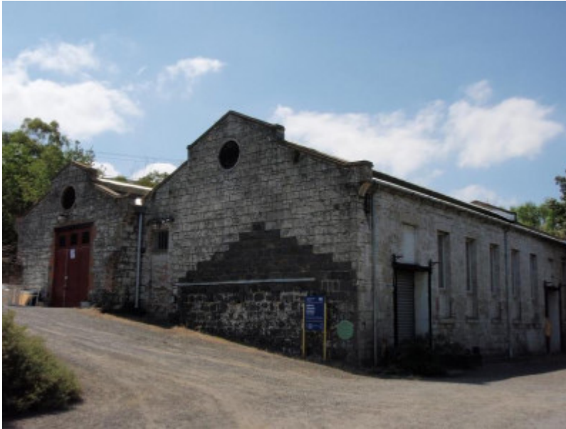
HO64(5) - Former Melbourne Meat Preserving Co. Pipemakers Park, Maribyrnong.JPG
