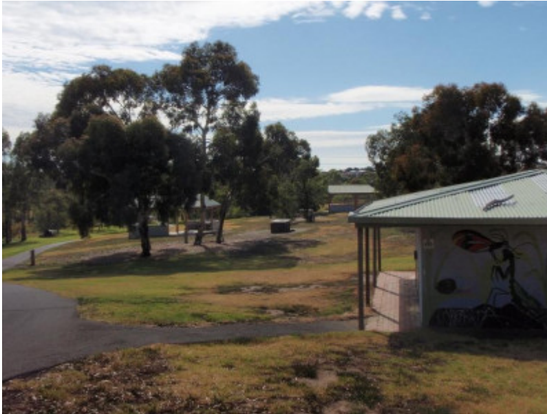
HO64(2) - Former Melbourne Meat Preserving Co. Pipemakers Park, Maribyrnong.JPG
