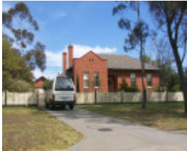
HO72(1) - Former Ordnance Factory, Wests Road, Maribyrnong.JPG
