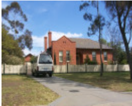
HO72(1) - Former Ordnance Factory, Wests Road, Maribyrnong.JPG
