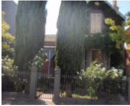
HO111 - James Darling House, 47 Cowper Street, Footscray.JPG
