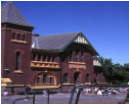
primary school number 2634 densham road armadale infant school side view
