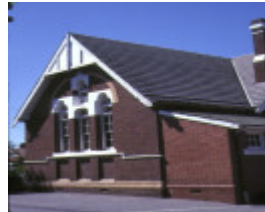
primary school number 2634 densham road armadale detail of front facade
