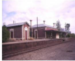
1 chiltern railway station & goods shed railway avenue chiltern trackside view apr1995
