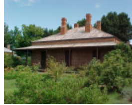
1 lakeview victoria street chiltern front elevation jan00
