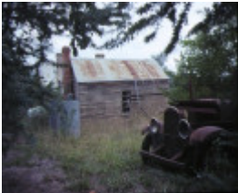
lakeview victoria street chiltern outbuildings may1981
