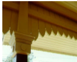
clayton railway station platform building detail sw nov1998
