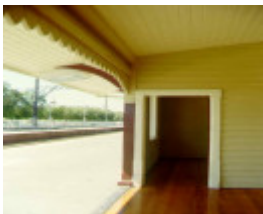
clayton railway station upside building sw nov1998
