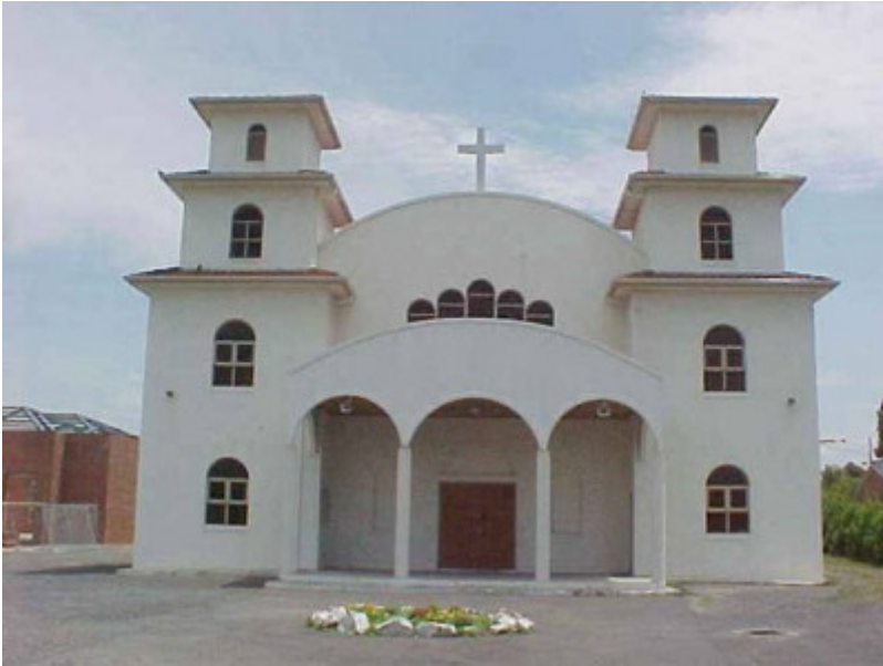
View from Amis Crescent
