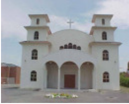
View from Amis Crescent
