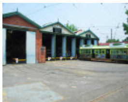
BENDIGO TRAM SHEDS, OFFICES AND POWER STATION SOHE 2008
