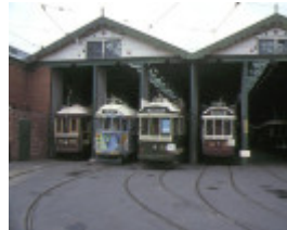
1 bendigo tram sheds front view of tram sheds
