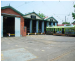
BENDIGO TRAM SHEDS, OFFICES AND POWER STATION SOHE 2008
