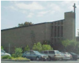
View of church from north side
