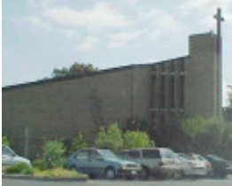
View of church from north side
