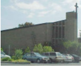
View of church from north side
