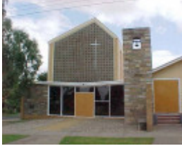
View of church from James Street
