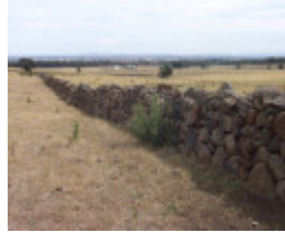
Dry Stone Wall R300
