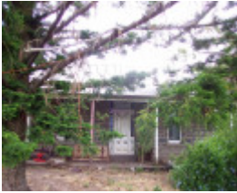
Glencoe (prior to renovation)
