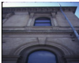
clunes post office detail exterior windows nov1984
