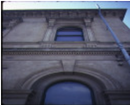
clunes post office detail exterior windows nov1984
