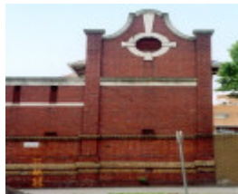
Northern Cattle Market Wall Flemington Rd
