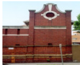
Northern Cattle Market Wall Flemington Rd
