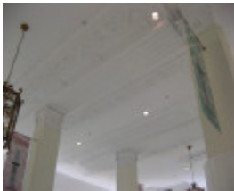
David Jones_plaster ceiling_16 Jan 08
