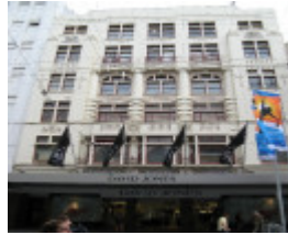
David Jones_1911 building & 1925 addition_16 Jan 08
