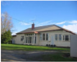
Valley View Orchards Managers House & Coolstore
