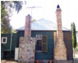
Paine's Cottage Chimneys
