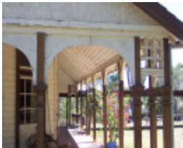
Cornwall Park Stud - verandah detail
