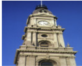
collingwood town hall clock tower detail jul1983
