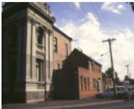
collingwood town hall rear view jul1983
