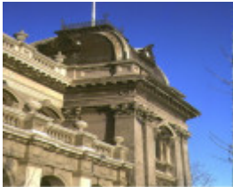
collingwood town hall balcony detail jul1983
