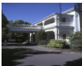
armadale house kooyong road armadale entrance jan1985
