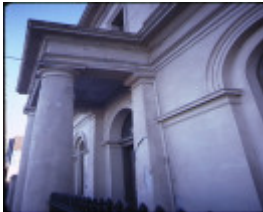
former es&a bank clunes front columns
