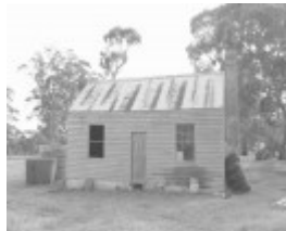
Workers' (probably shearers') quarters behind shearing shed.
