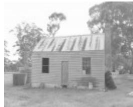
Workers' (probably shearers') quarters behind shearing shed.
