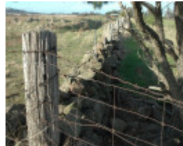
Dry Stone Wall R193
