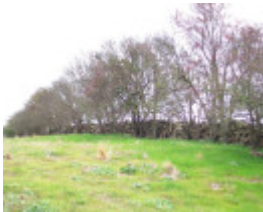
Dry Stone Wall R6
