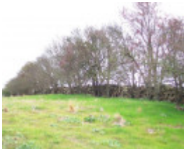
Dry Stone Wall R6
