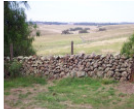
Dry Stone Wall R6
