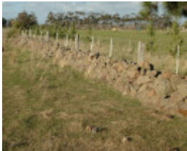
Dry Stone Wall R193
