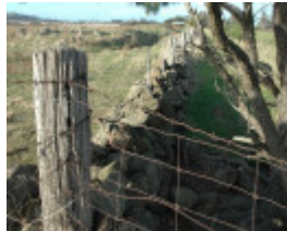
Dry Stone Wall R193
