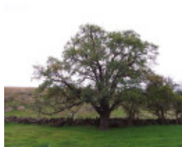
Dry Stone Wall R6
