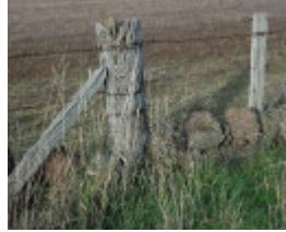
Dry Stone Wall R248 - Black Hill Road Boundary
