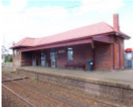
Railway Station and Platforms (pre-upgrade for metropolitan rail service)
